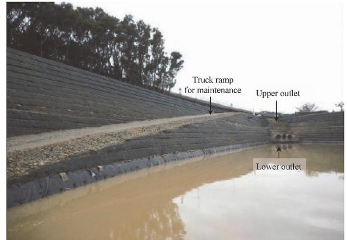
Fig. 9 Detention pond with outlets, reinforced soil slope and downslope ramp for truck access
