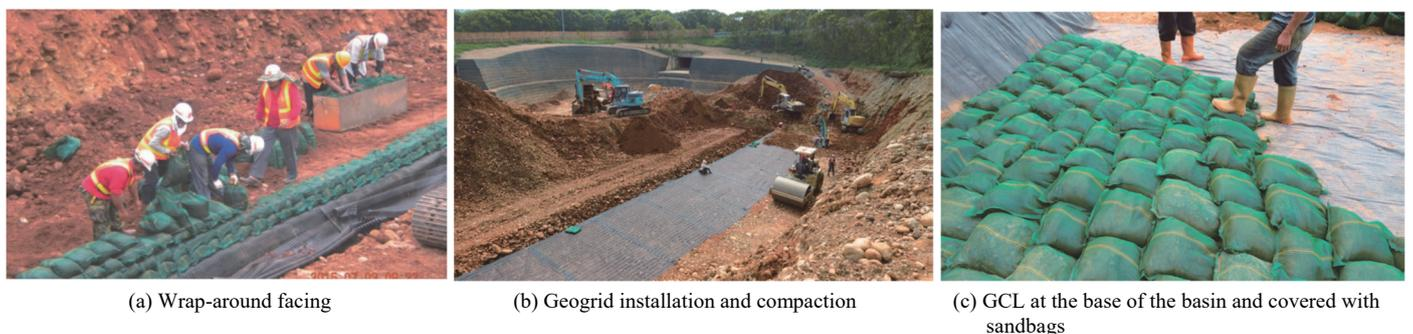
Fig. 11 Construction details
