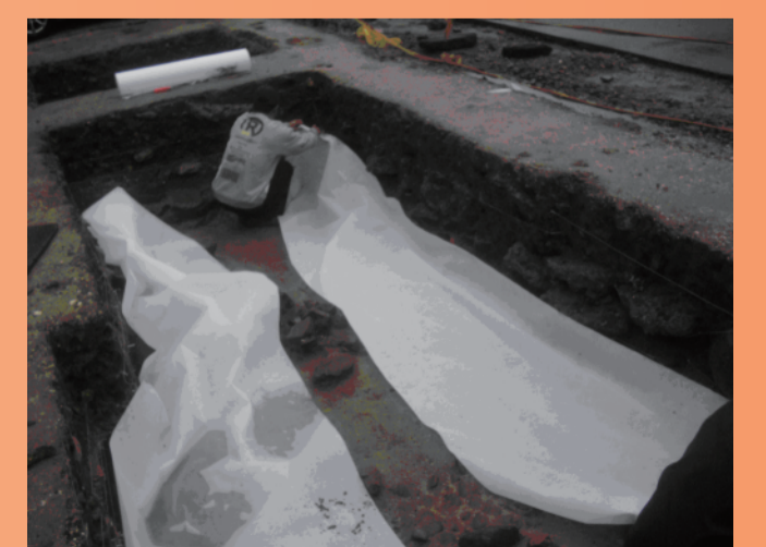
Photo 15: Covering the rammed earth
