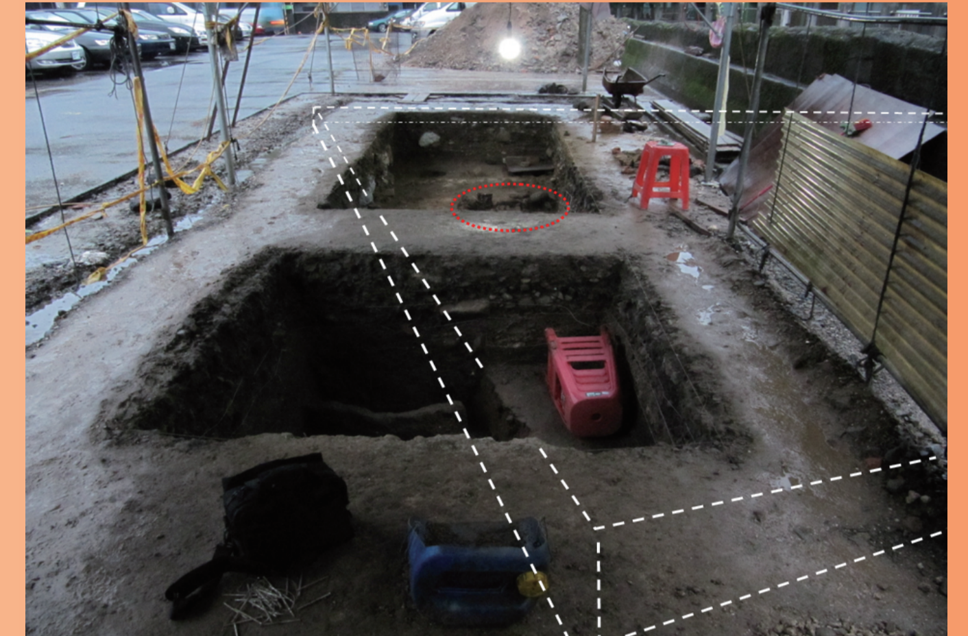
Photo 14: Test-pits 4 & 5-6 (combined in a single one), showing the rammed earth.
