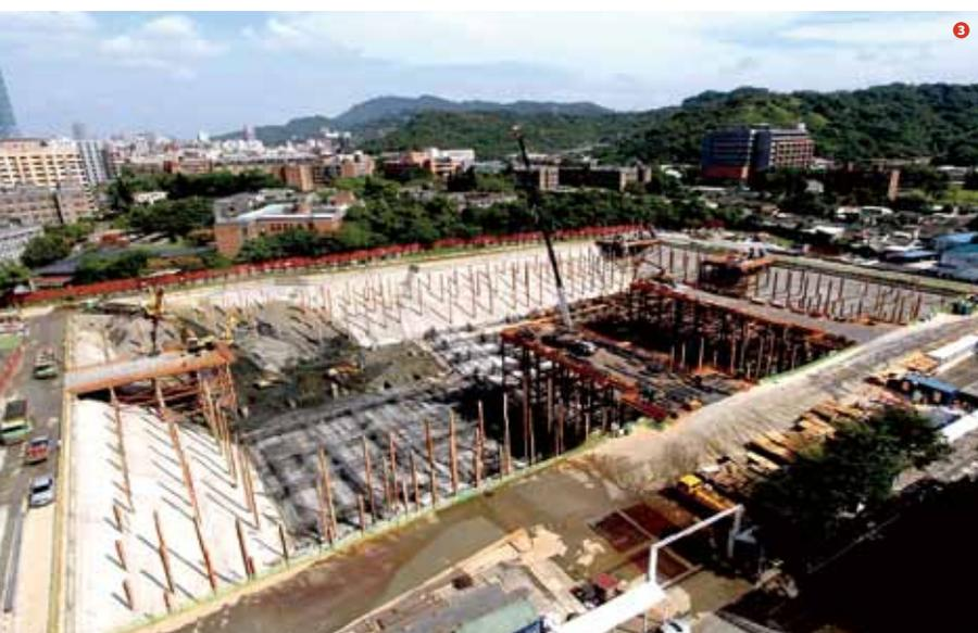
3 The construction team has created the hospital's subterranean levels through an approach called island excavation.
