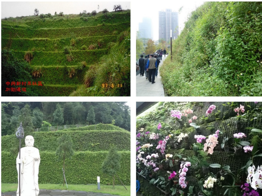
Fig. 15 Typical geogrid-reinforced walls with the wrap-around facings in Taiwan. The geogrids allow grass to grow through the grid
