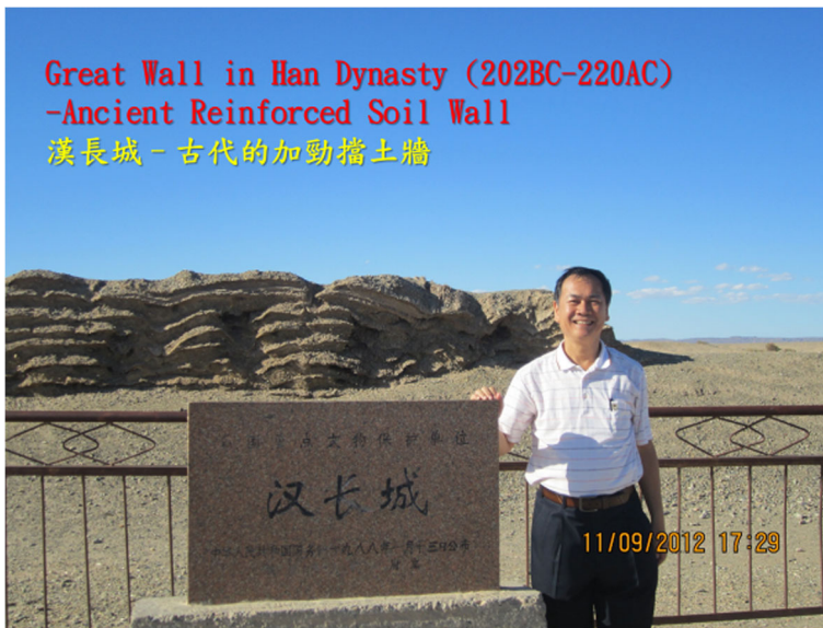
Fig. 2 The Great Wall of the Han Dynasty in Yangguan Pass, China, an ancient reinforcing soil structure
