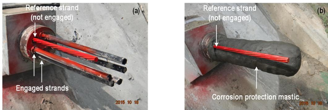
Fig. 7. The photo of a sensing anchor during installed: (a) reference strand and engaged strands and (b) engaged strands and anchor head protected with mastic.
