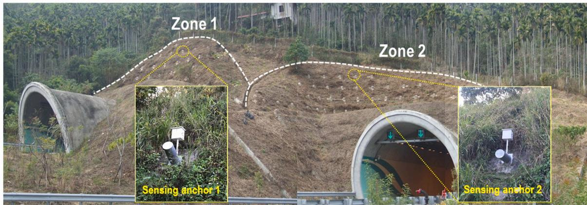
Fig. 6. Perspective view and sensing anchors in an anchored slope (freeway-side 6 in central Taiwan).
